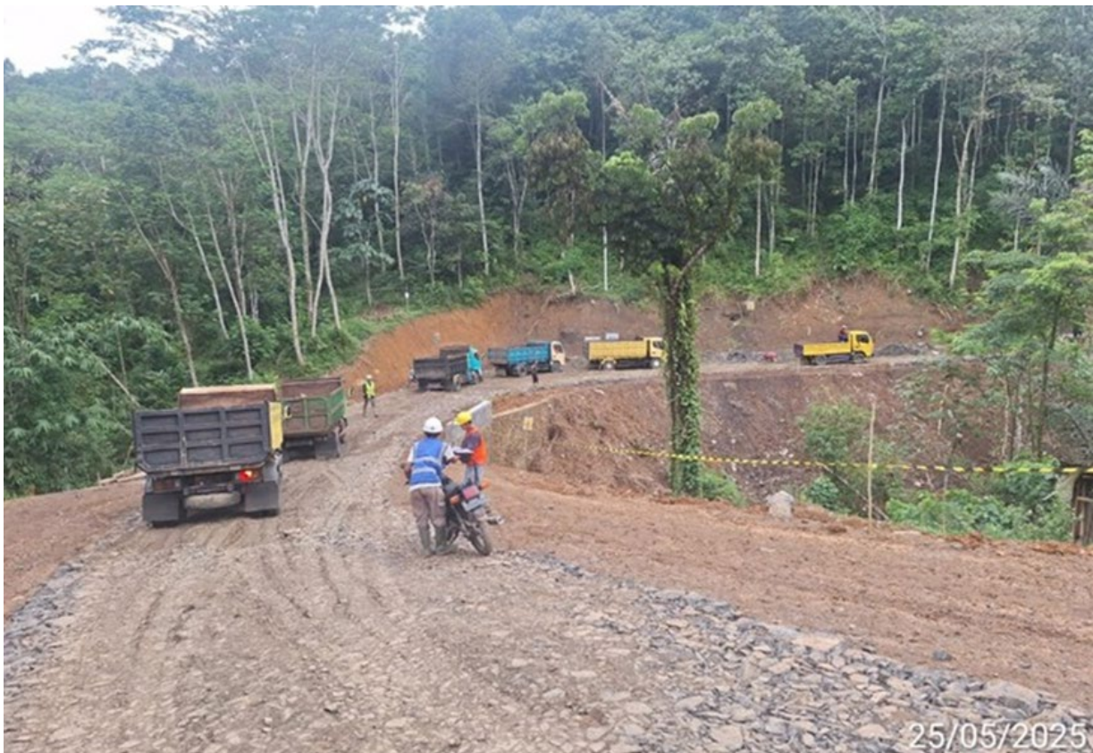
Nagajaya, Indonesia, Access road
